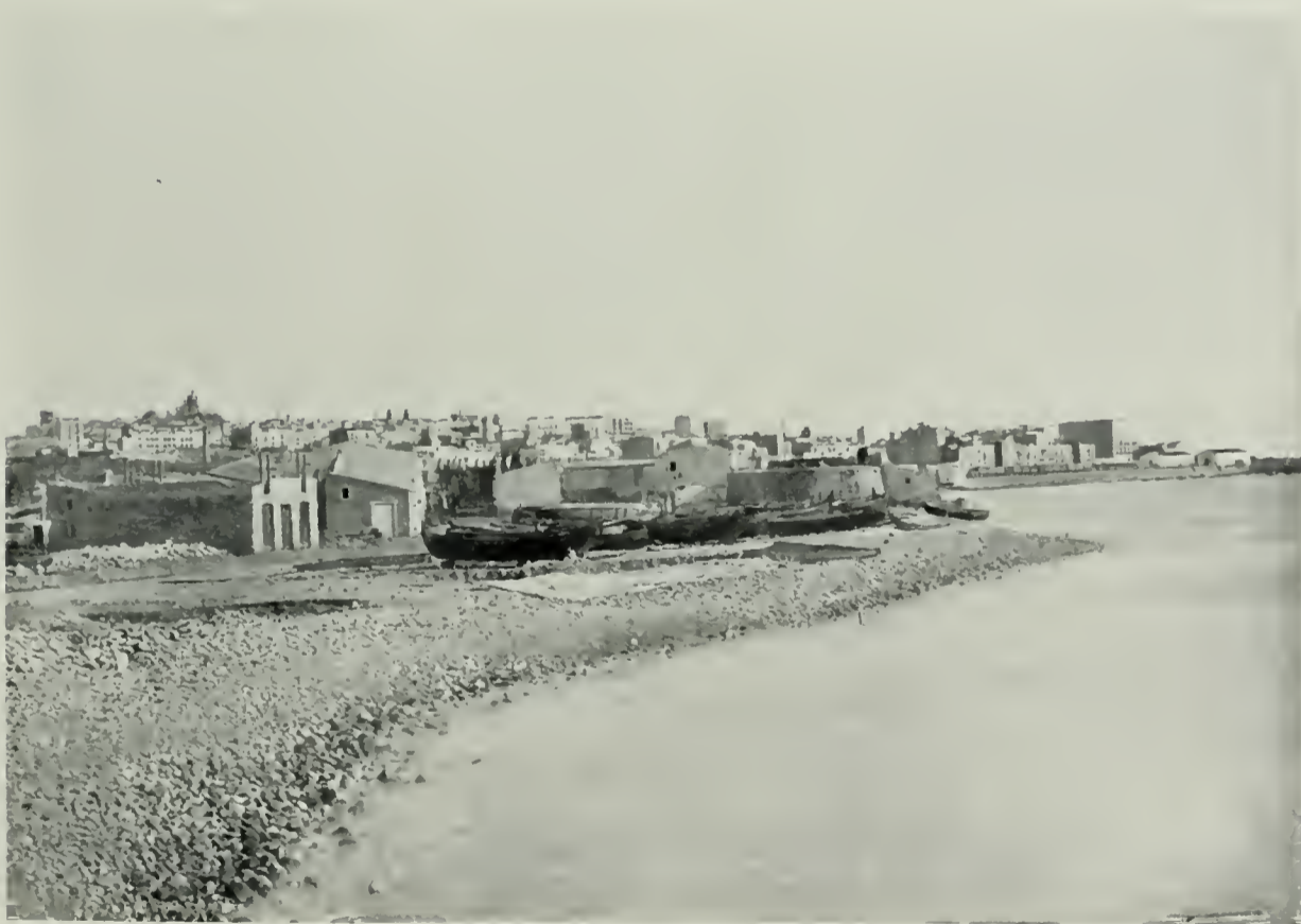
GENERAL VIEW OF TARRAGONA
